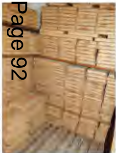
Unconditioned storage in the east end.
