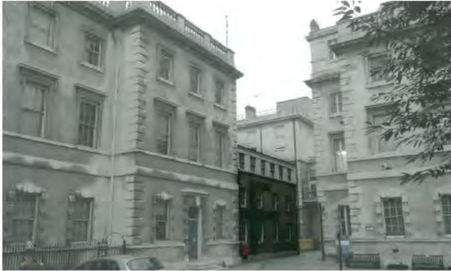
North Wing with Existing Extension
