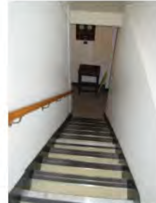
Existing stairs to WCs in the West End are really too narrow (790mm) for public access. Under the Insall/Maggle's scheme these stairs will become the main access route to the public WCs in the West end Basement, remote from the main Hogarth Entrance
